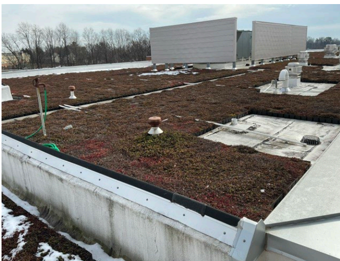
9 - TPO ROOF WITH GREEN ROOF
