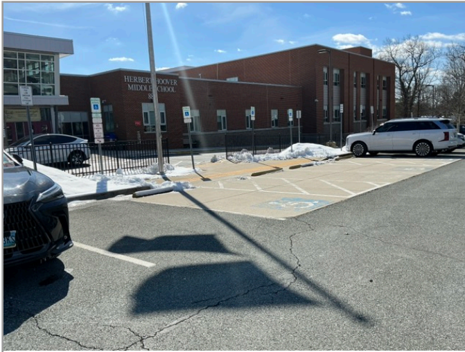
OVERVIEW OF ACCESSIBLE PARKING AREA
