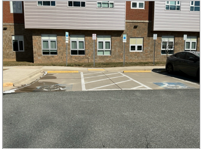
2ND AREA OF ACCESSIBLE PARKING
