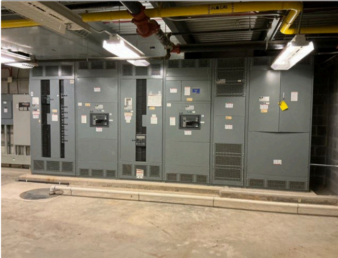
25 - MAIN SWITCHGEAR
